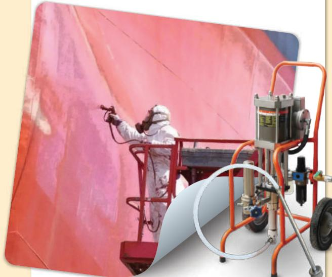
It is engineered for use across shipbuilding, steel structure fabrication, offshore facilities, railway maintenance, heavy machinery, and industrial infrastructure. This equipment excels in the application of modern protective coatings and thick-film, heavy-duty anti-corrosive systems, especially where conventional spraying methods may be insufficient or inefficient.
